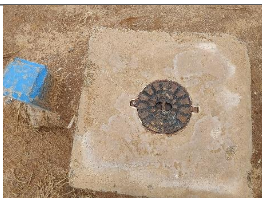
Photo No. 2.3.3-8: Close view of the water supply beacon and sewer manhole
