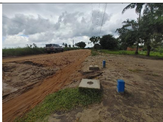
Photo No. 2.3.3-7: Water supply pipeline and sewer manhole at km on the road median at km 0 + 829.
