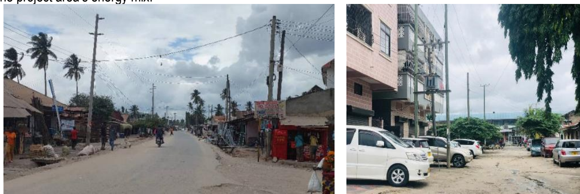
Figure 4-8: Electricity line along one of the proposed roads
