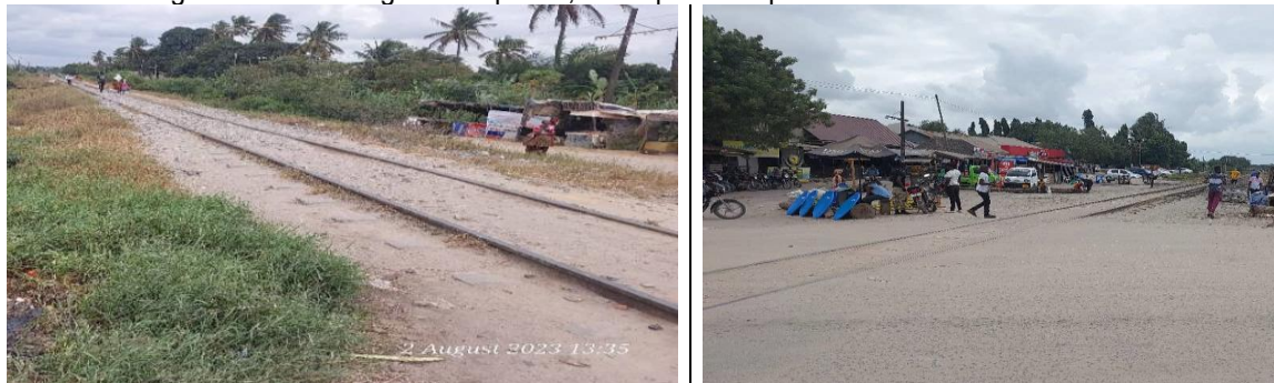
Figure 4-6: Railway crossing Kitunda-Kivule-Msongola road
