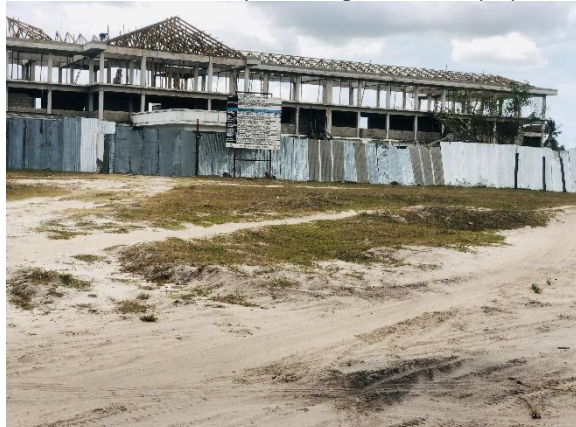
Kivule District Hospital under construction along /Kivule-Majohe Jct road
