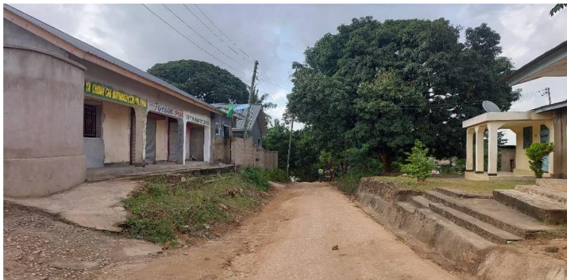
Figure 6-1: House extension and verandas along the Migombani road that the project could impact
