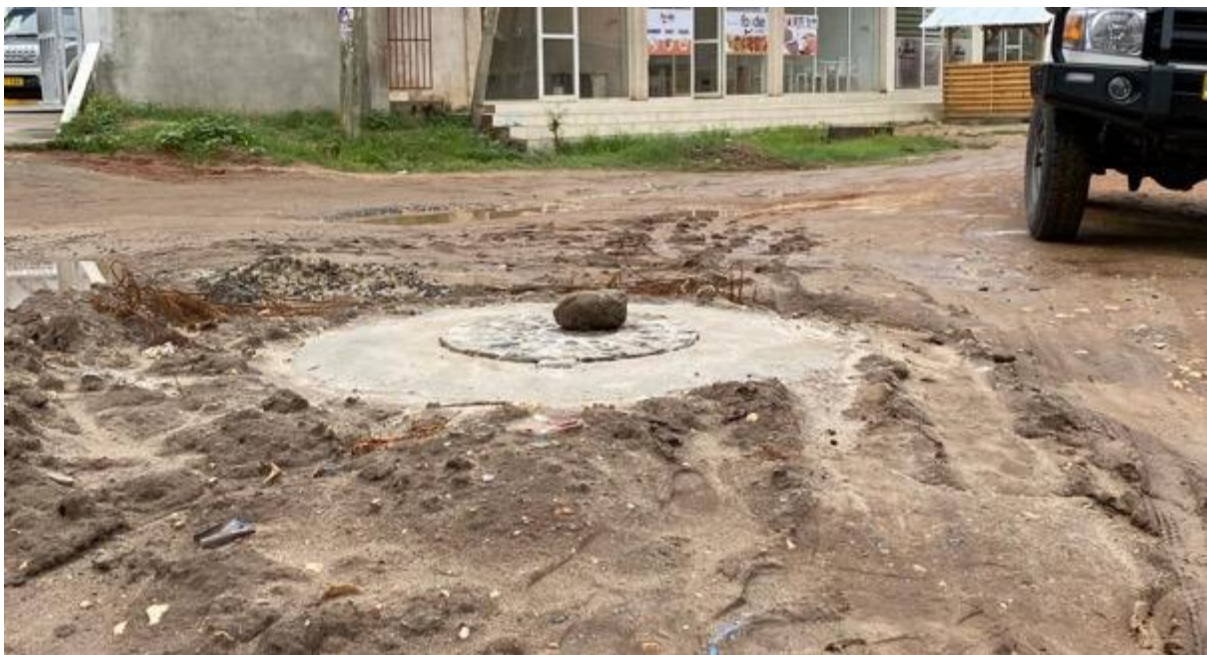
Figure 2-61: Newly Constructed Sewerage System Manhole at Km 0 + 100 Sheikh Bofu Road
