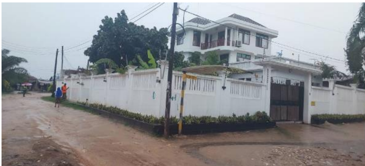
Figure 2-111: One of the Houses whose Fence will be Partially Demolished, Photo Taken at Km 0+030 LHS of Mikindani Road
