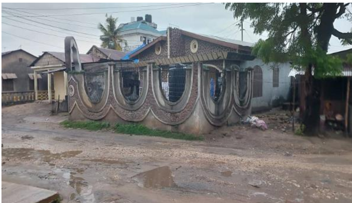
Figure 2-157: Narrow Corridor at Km 0+320 of Binti Kayenga Road, a House whose Fence will be Demolished
