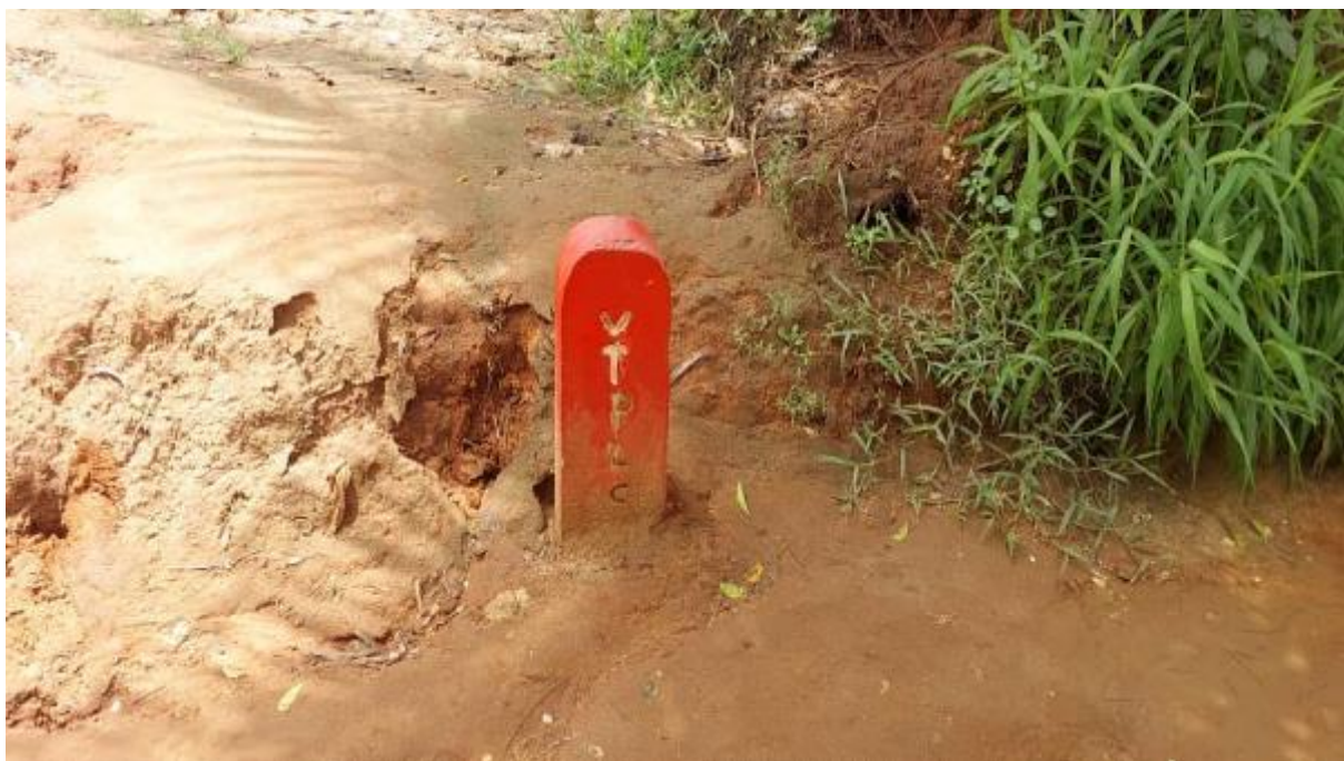
Figure 2-18: A Concrete Marker Post for Telecommunication Cable found at Km 2 + 065 LHS of the Proposed Msumi Road
