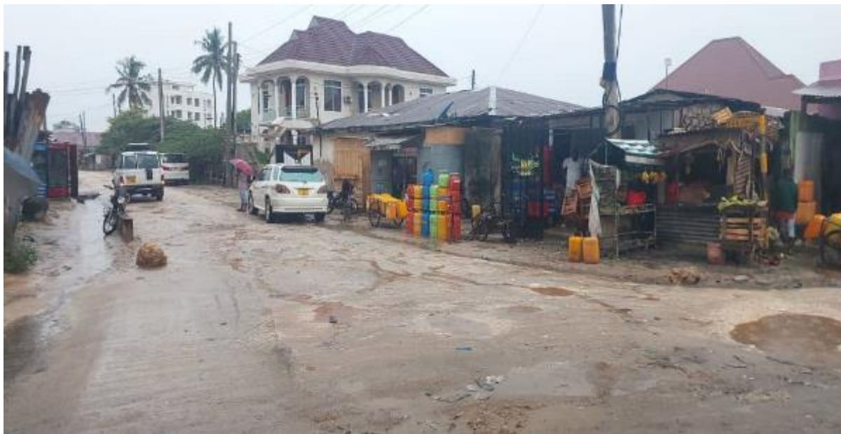
Figure 2-111: Starting Point of Chimwaga Road, forms T-Junction with Namnani Road
