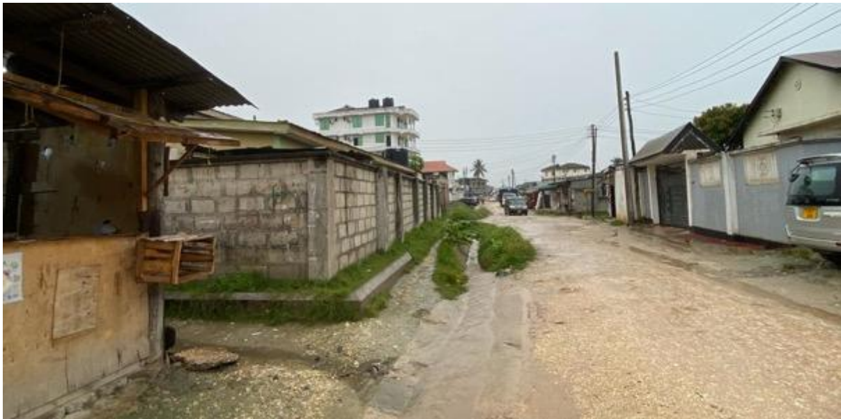
Figure 2-113: One of the Houses found at Km 0+100 LHS whose Fence will be Demolished
