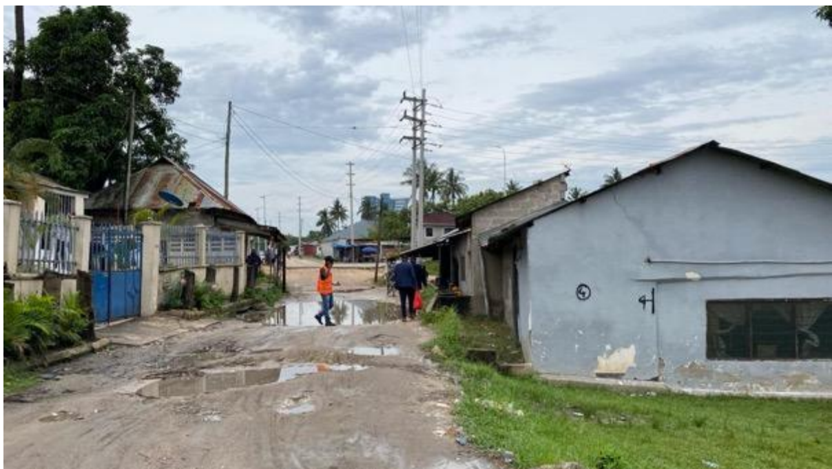
Figure 2-131: Narrow Corridor at Km 0+350 LHS of Ubungo NHC Road
