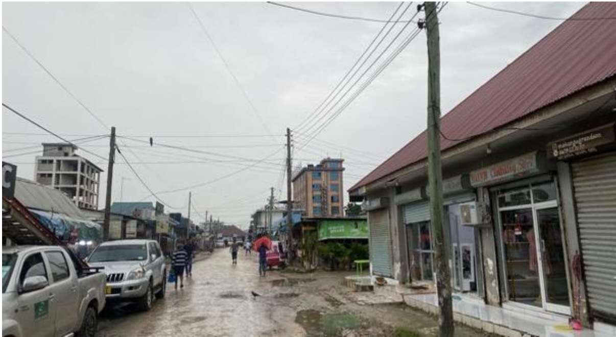
Figure 2-99: Shops and Traffic Condition at Km 0+000 of Namnani Road
