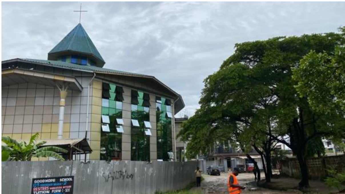
Figure 2-130: A TAG Church found at Km 0+100 LHS of Ubungo Spur NHC Road
