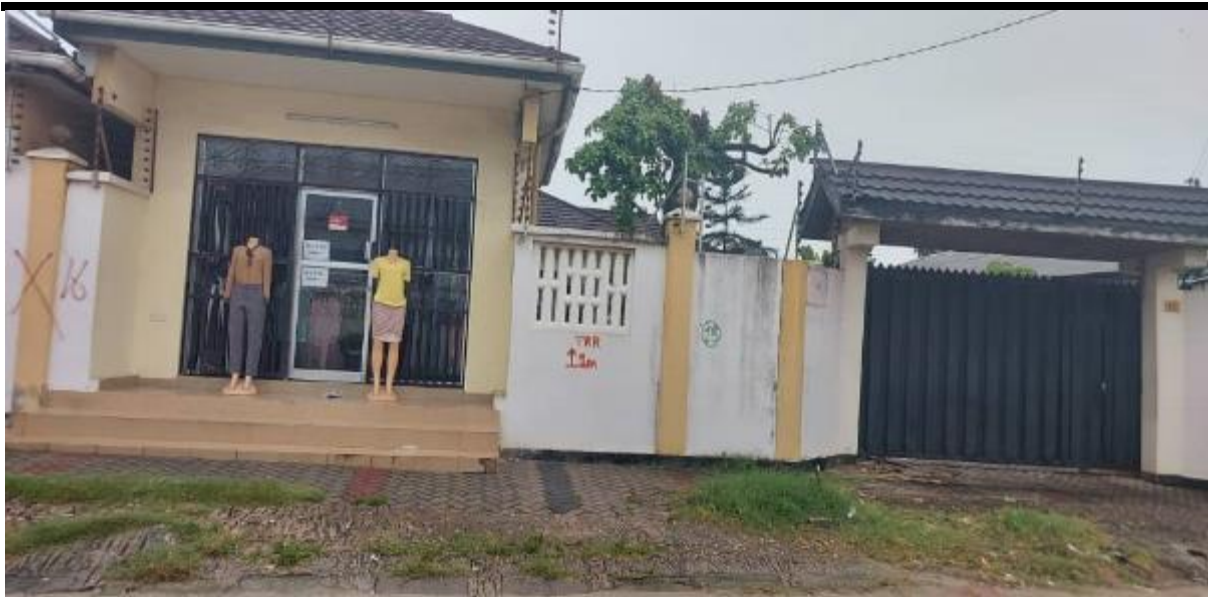
Figure 2-91: One of the Houses which will be Partially Demolished, Photo Taken at Km 0+580 LHS of Juma Ikangaa Road
