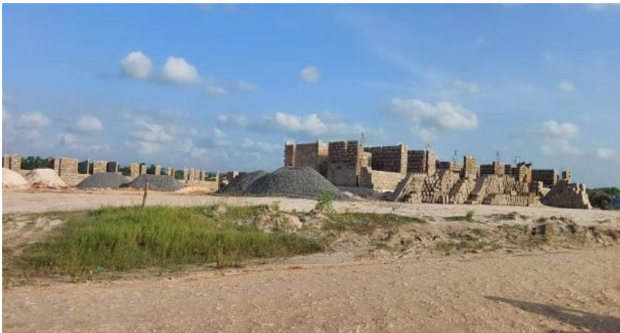
Figure 2-44: VETA Buildings under Construction at Km 2 + 970 RHS of the Proposed Hondogo Shija Road
