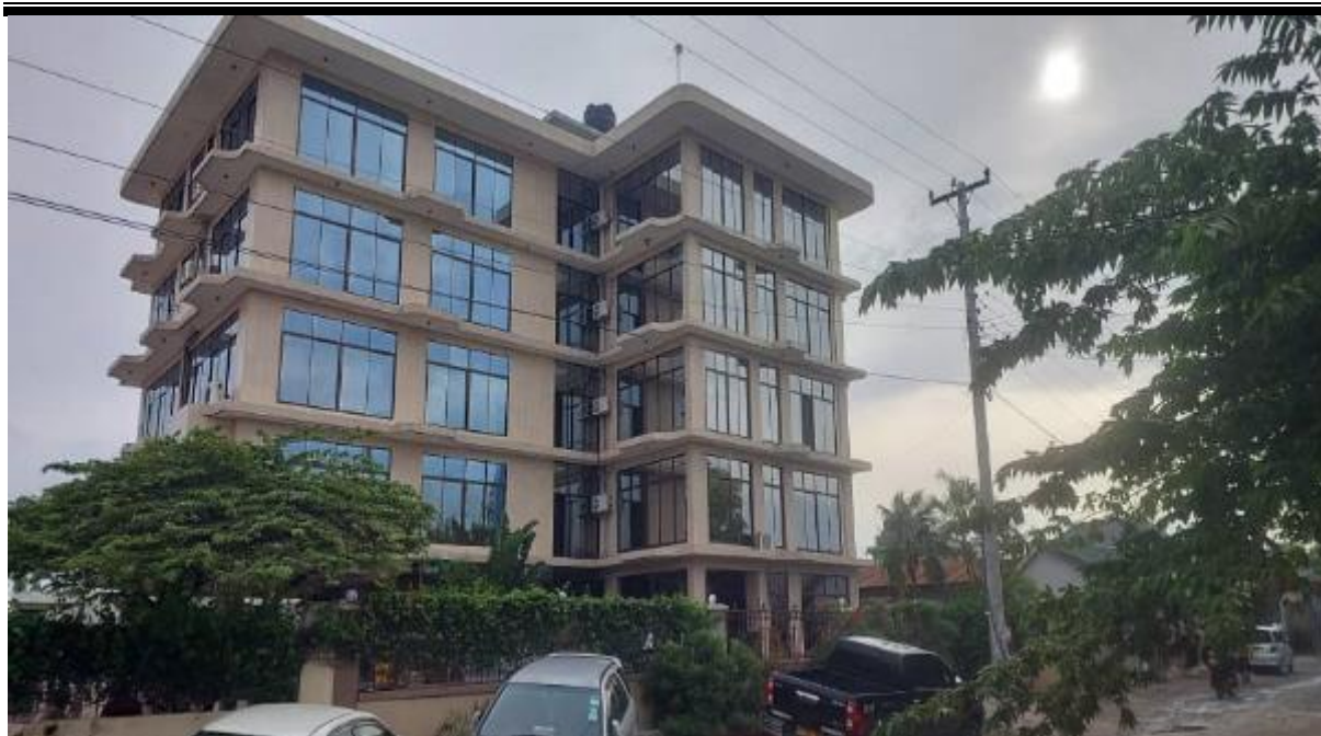
Figure 2-73: Hotel Building found at Km 0+070 RHS of Sinza KKKT Road
