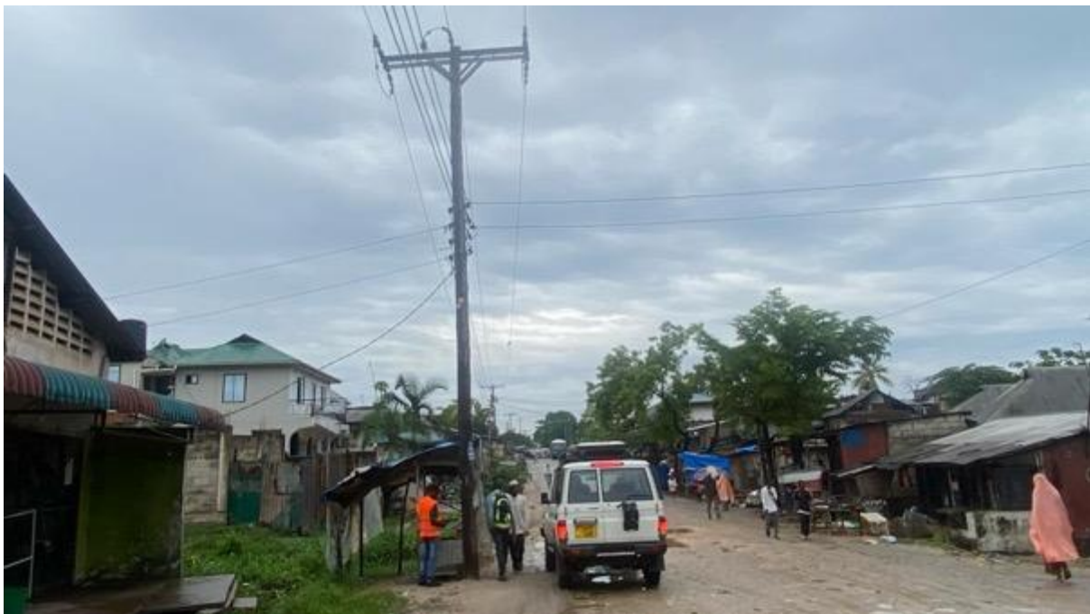
Figure 2-148: 13kV Electric Power Line found at Km 0+400 LHS of Midizini Road
