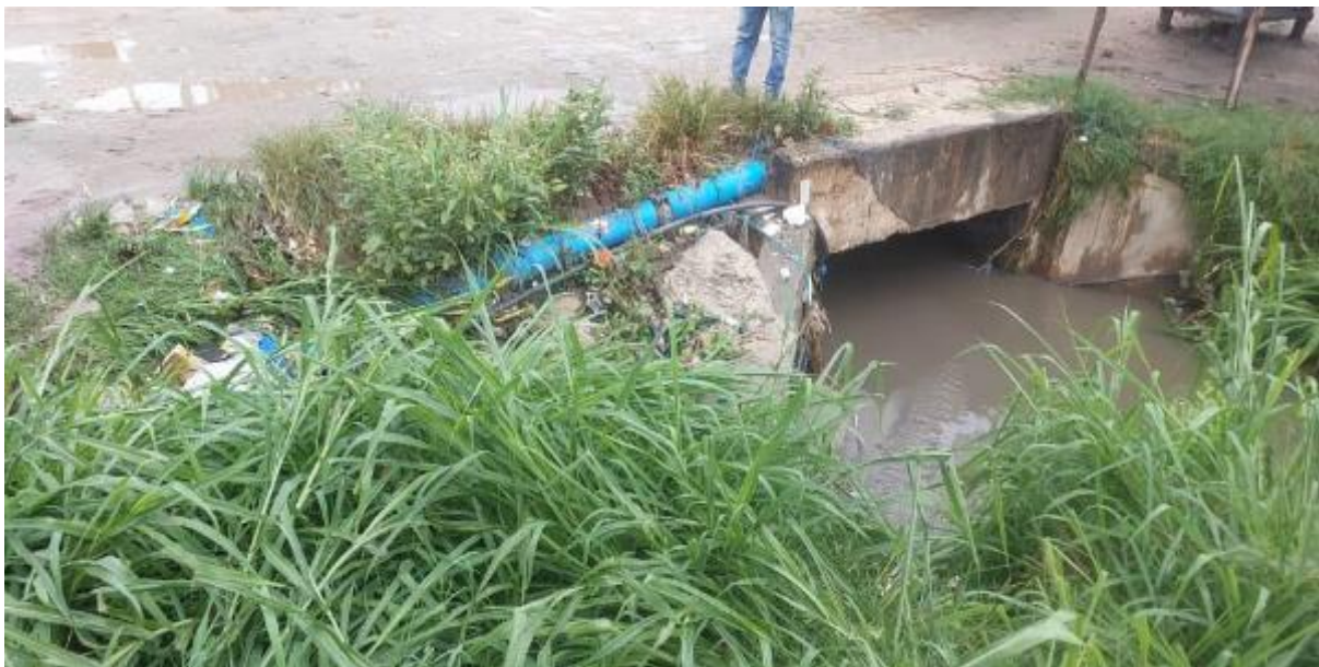
Figure 2-150: Water Supply Pipelines Crosses China River at Km 0+400 LHS of Midizini Road
