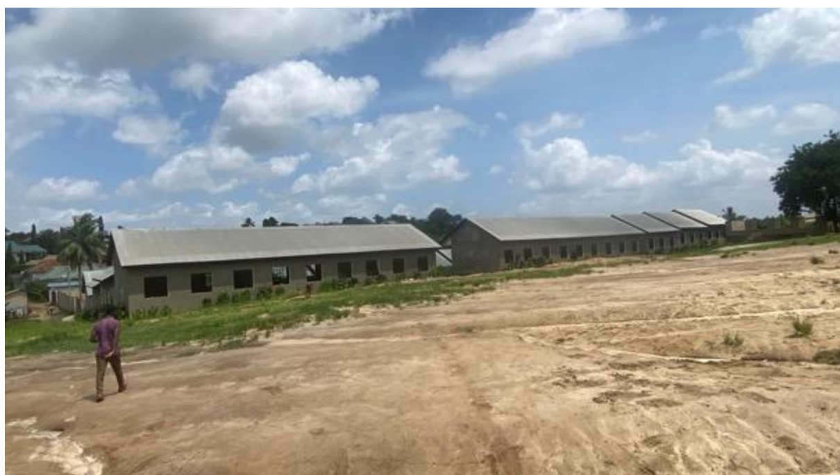
Figure 2-12: Makabe Secondary School Located at Km 4 + 700 RHS of the Proposed Msumi Road
