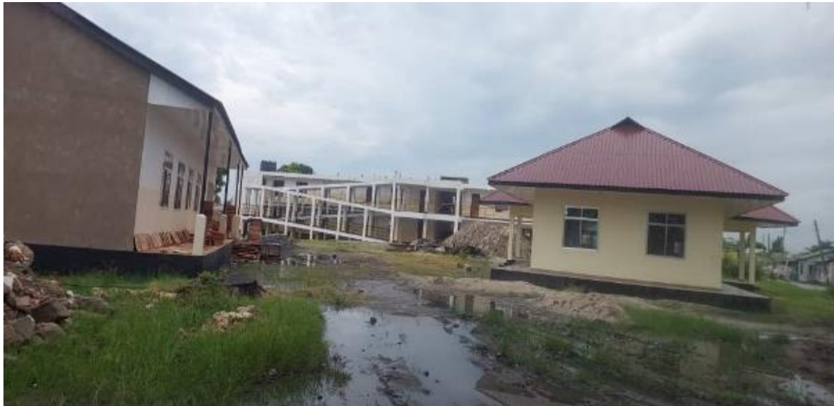
Figure 2-126: Ubungo Secondary School found at Km 0+000 RHS of the Ubungo NHC Road Source: Field Survey by the Consultant (June 2023)
