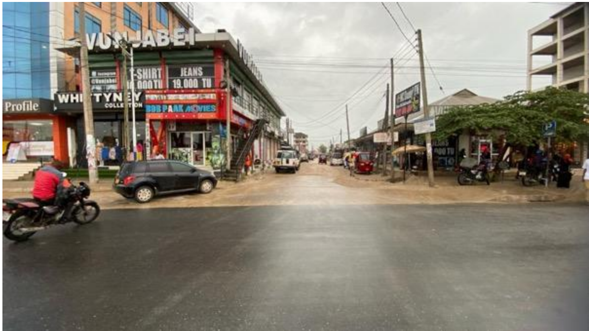
Figure 2-95: Starting Point of Proposed Namnani Road, at intersection with Shekilango Road Source: Field Survey by the Consultant (June 2023)
