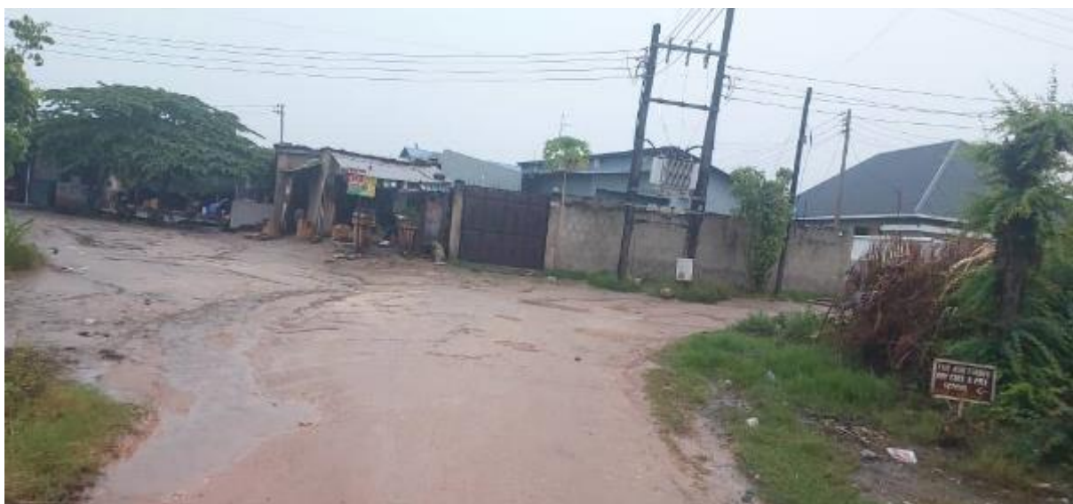
Figure 2-106: Electric Power Substation found at Km 0+280 RHS of Mbegani Road
