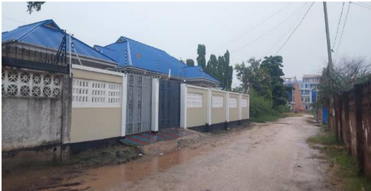
Figure 2-107: A Typical Residential House found at 0+500 LHS along Shule Road Source: Field Survey by the Consultant (June 2023)
