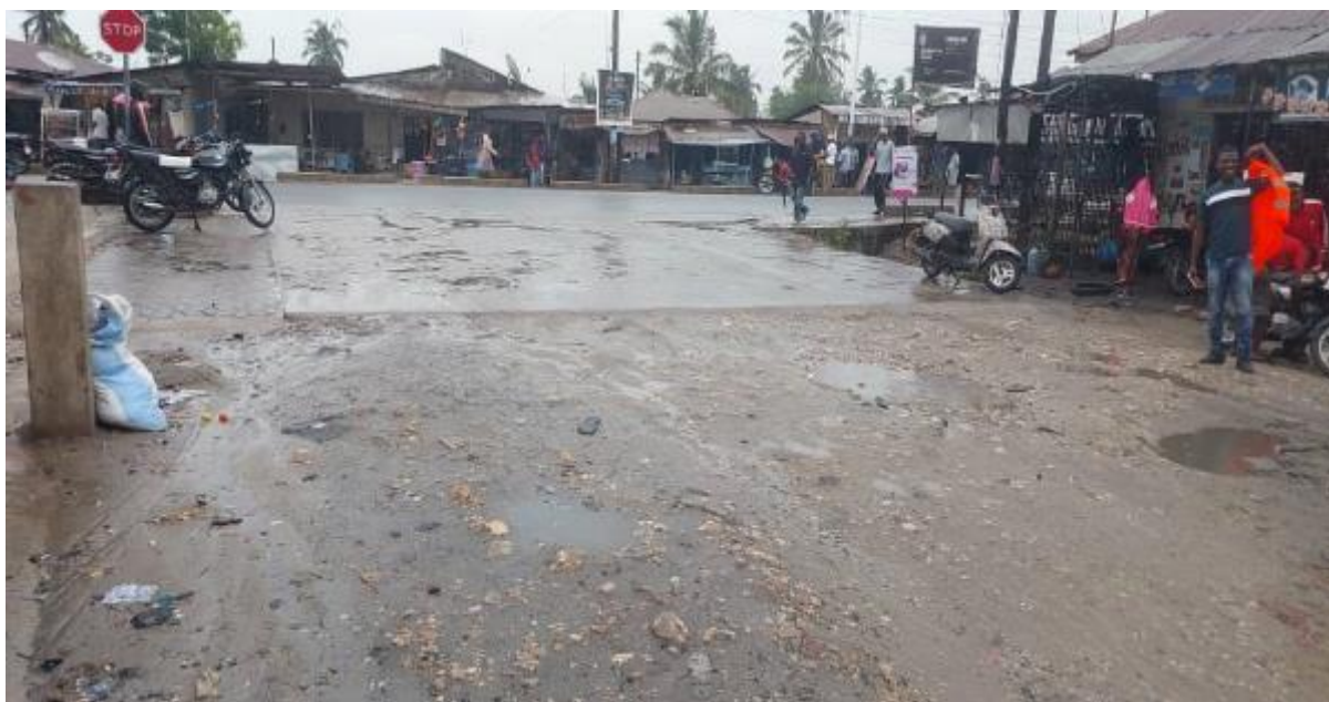
Figure 2-134: Starting Point of Tiptop Road, at T-Junction with Mabibo – Mburahati Road
