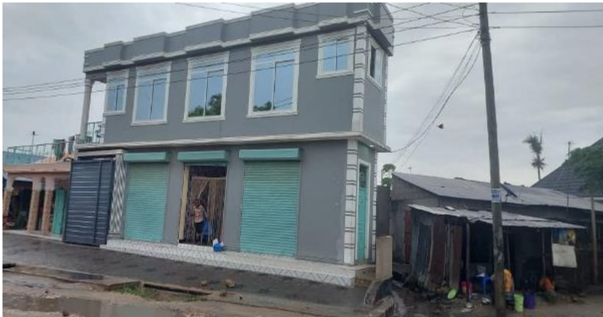
Figure 2-155: Commercial Building found at Km 0+310 RHS of Binti Kayenga Road Source: Field Survey by the Consultant (June 2023)
