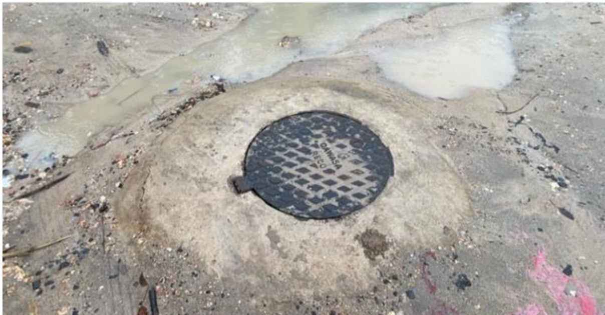
Figure 2-122: Sewer Manhole found at Km 0+700 within Construction Corridor of Lion Road Source: Field Survey by the Consultant (June 2023)
