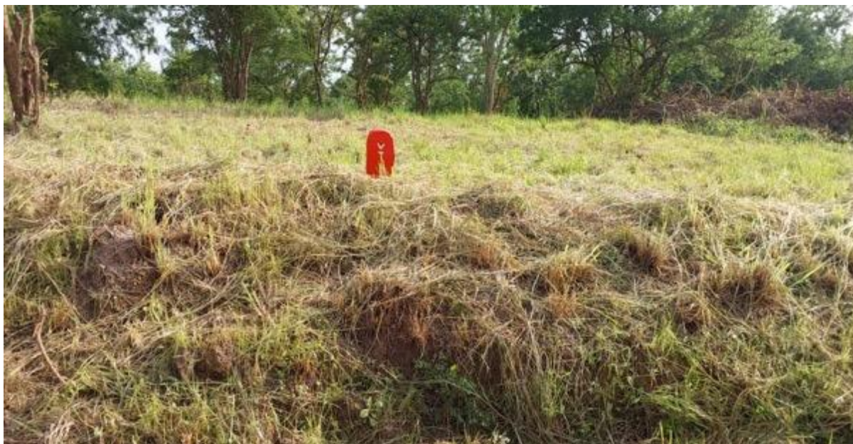
Figure 2-49: A Concrete Marker Post for Telecommunication Cable found at Km 0 + 600 RHS of the Proposed Hondogo Shija Road
