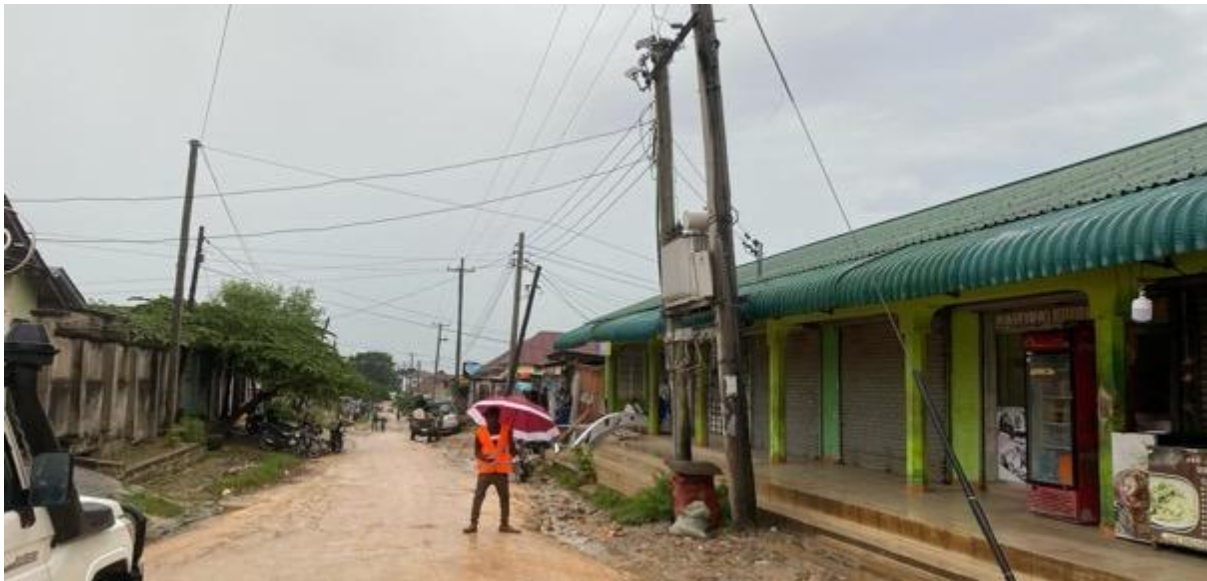
Figure 2-101: 33kV Electric Power Substation found at Km 0+350 LHS of Namnani Road
