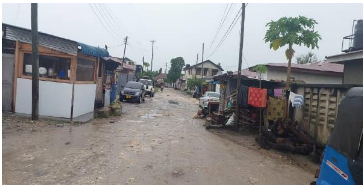
Figure 2-93: Electric Poles found at Km 0+070 of Juma Ikangaa Road
