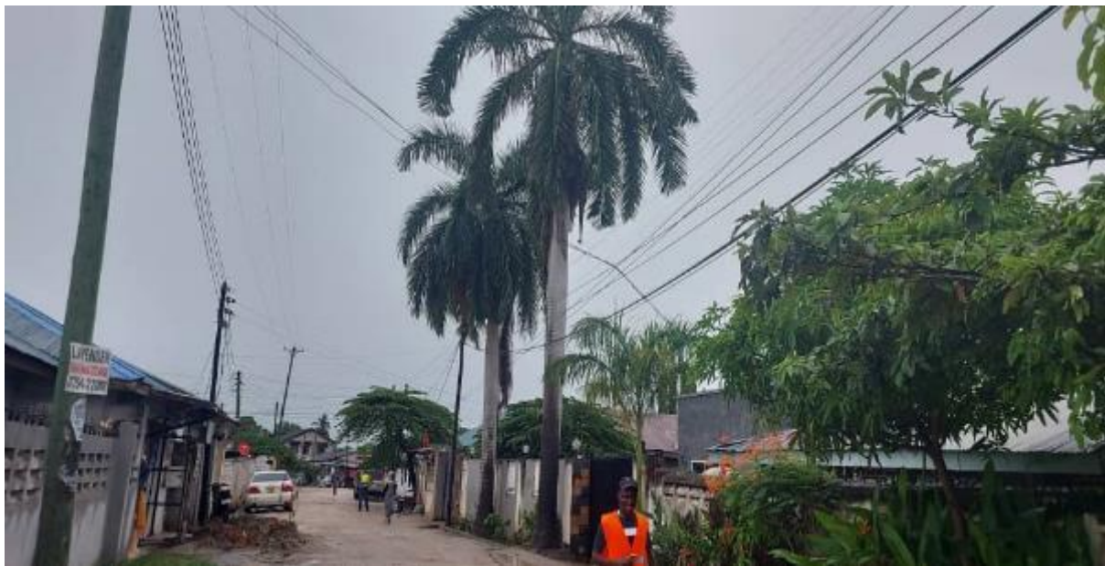
Figure 2-92: Palm Trees and Houses found within Construction Corridor at 0+115 of Juma Ikangaa Road
