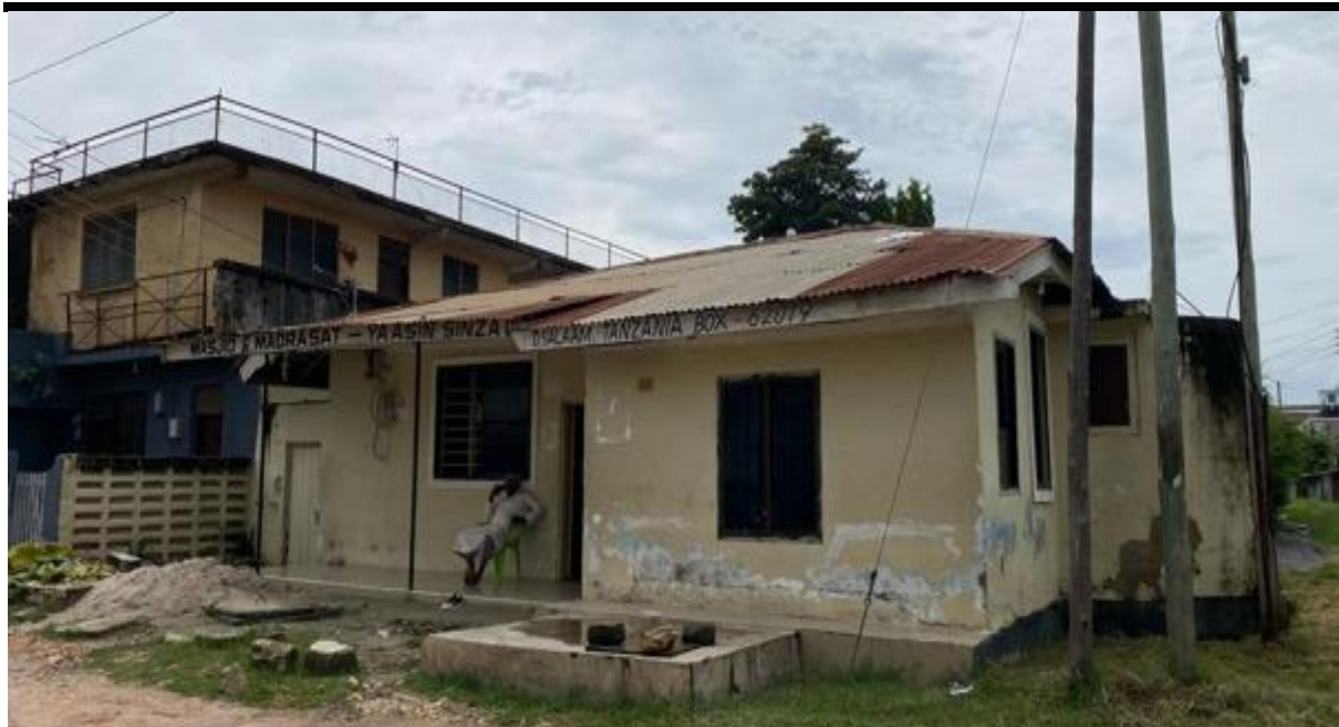
Figure 2-56: Masjid and Madrasa found at Km 0+800RHS of Sheikh Bofu Road
