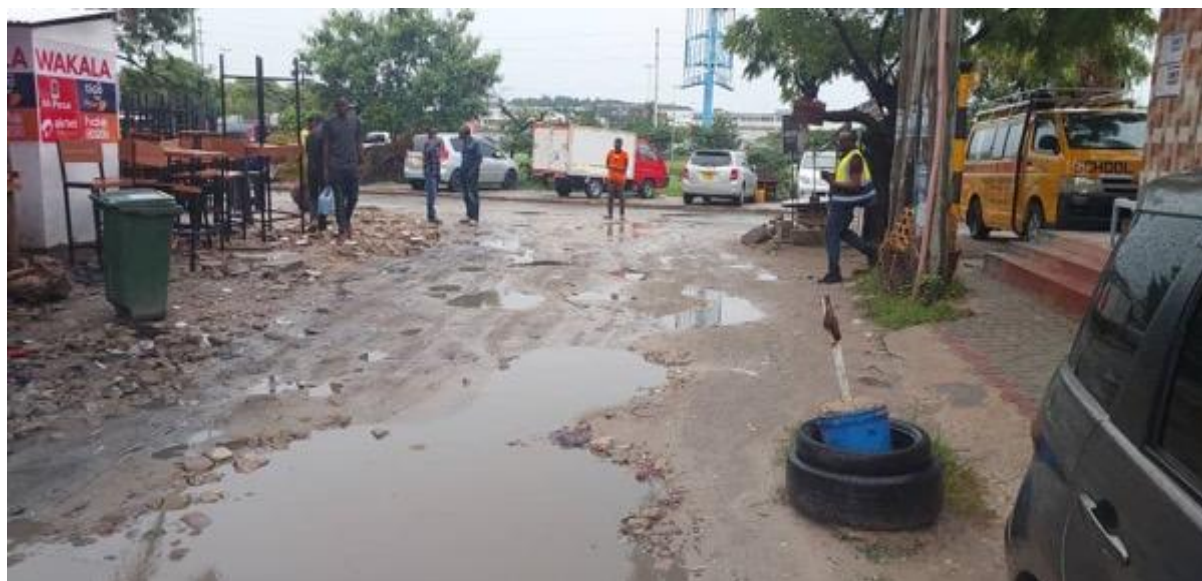
Figure 2-77: Starting Point of Segesera Road, at T-Junction with Sum Nujoma Road
