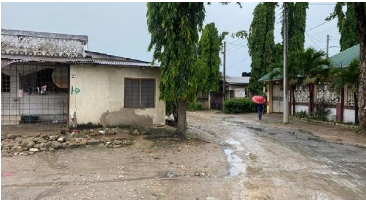
Figure 2-100: One of the Houses to be Demolished at Namnani Road, Photo Taken at Km 0+250 LHS
