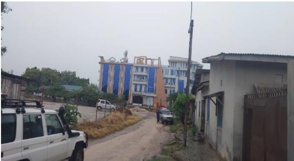
Figure 2-110: An Electric Pole found at Km 0+200 RHS of Shule Road Source: Field Survey by the Consultant (June 2023)
