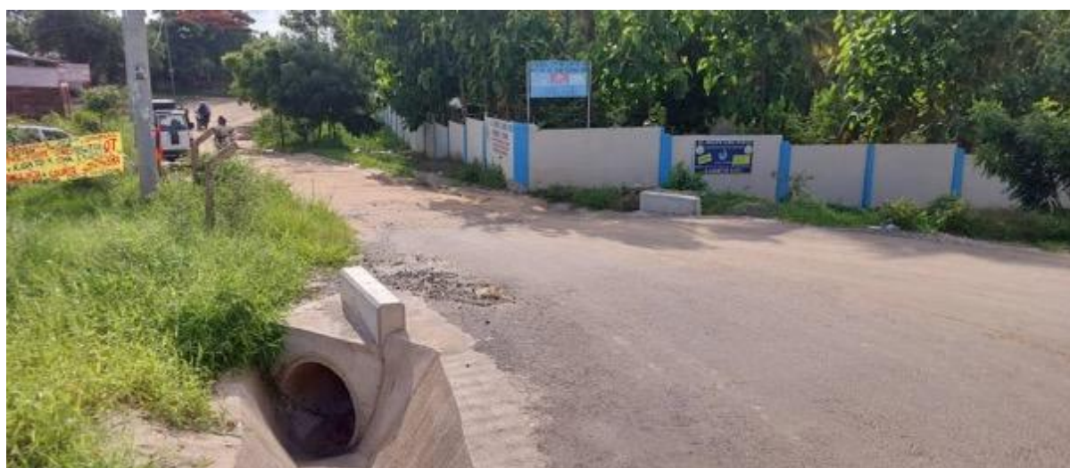
Figure 2-39: Start of Hondogo Shija Road at Junction of Kibamba Shule Road, Wall on LHS is the Rehabilitation Centre for Victims of Trafficking Girls
