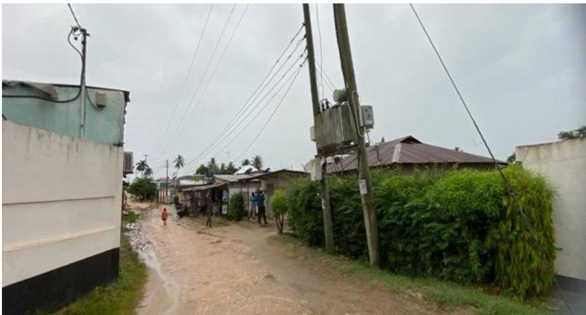
Figure 2-102: Starting Point of Mbegani Road, at Intersection with Namnani Road
