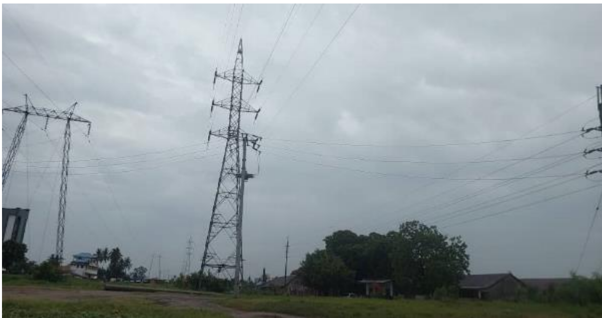
Figure 2-137: High Tension 400kV Power Line Crossing Tiptop Road
