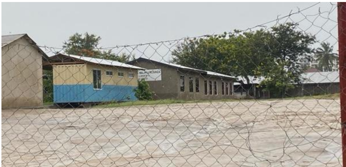
Figure 2-105: Sinza Primary School found at Km 0+200 LHS of the Shule Road
