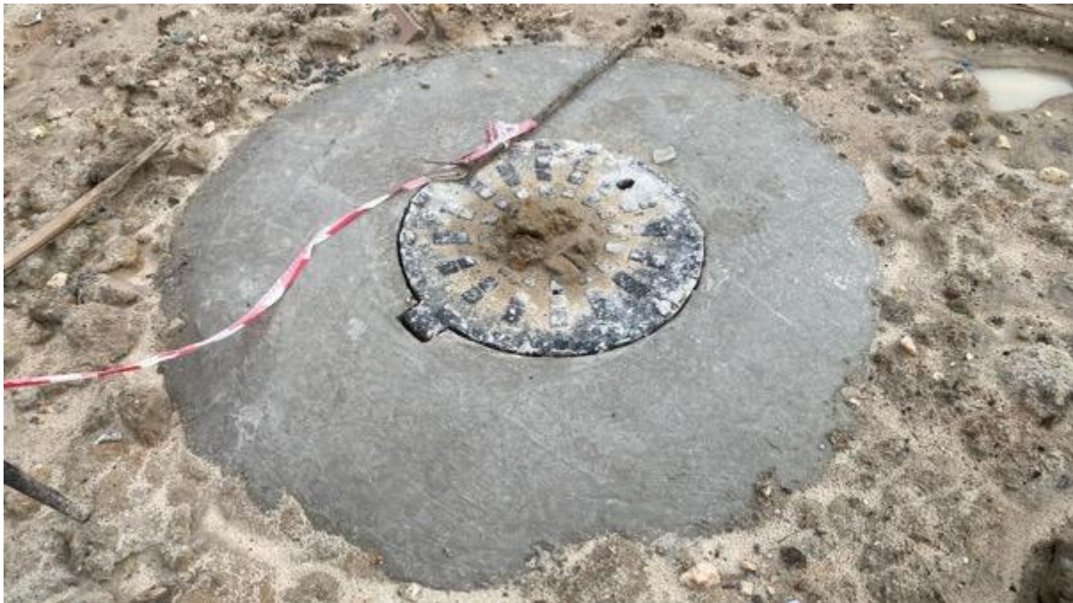
Figure 2-68: Newly Constructed Sewerage System Manhole at Km 0 + 070 of Msikitini Road
