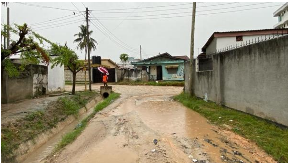
Figure 2-108: End of Mikindani Road, a T-Junction with Chimwaga Road
