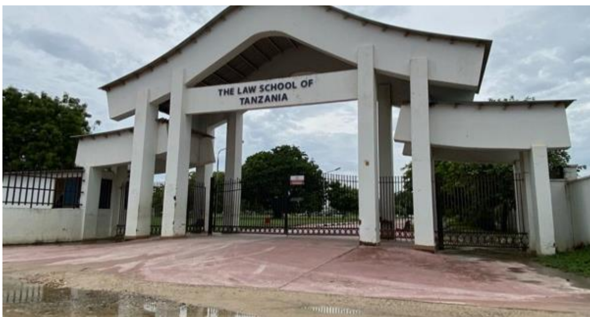
Figure 2-50: Entrance Gate of the Law School of Tanzania found at Km 0+200 LHS
