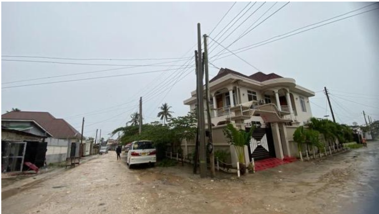
Figure 2-115: Electric Poles at Km 0+020 RHS of Chimwaga Road which are found within Construction Corridor
