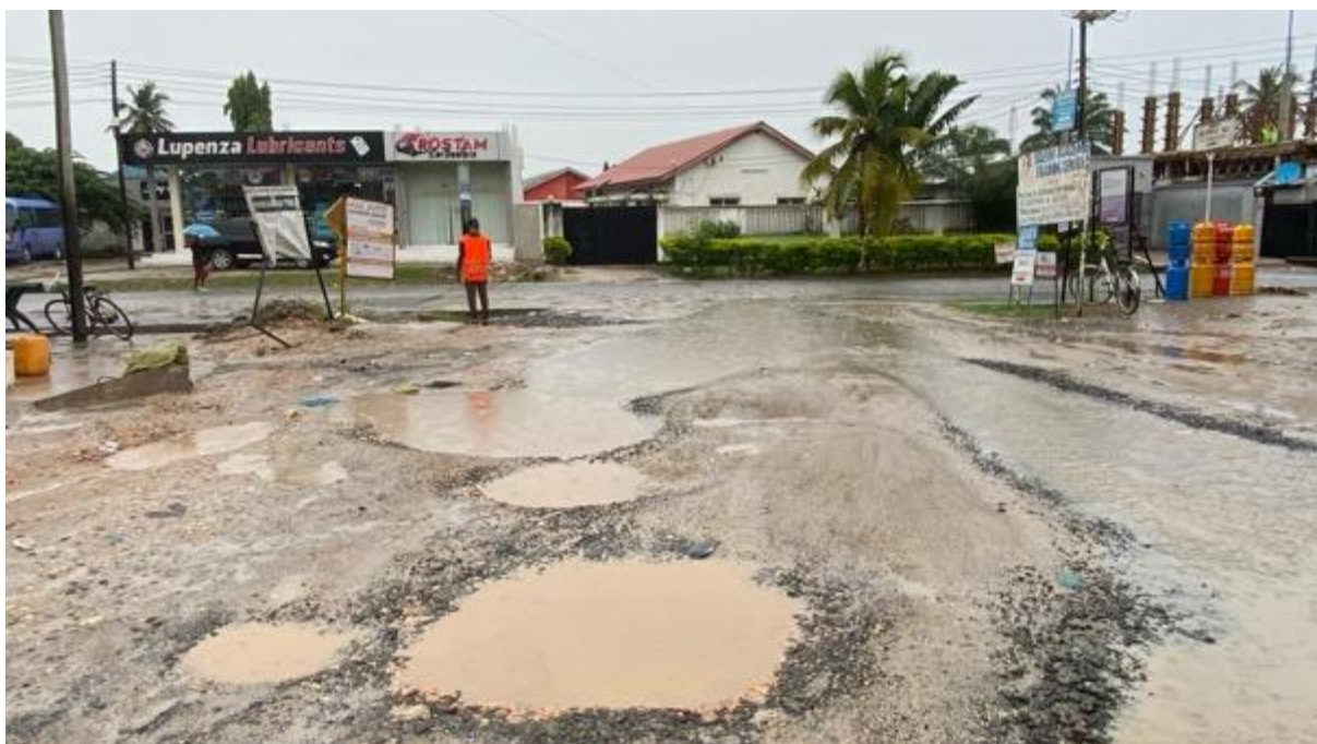
Figure 2-117: End of Lion Road, a T-Junction with Mori Road
