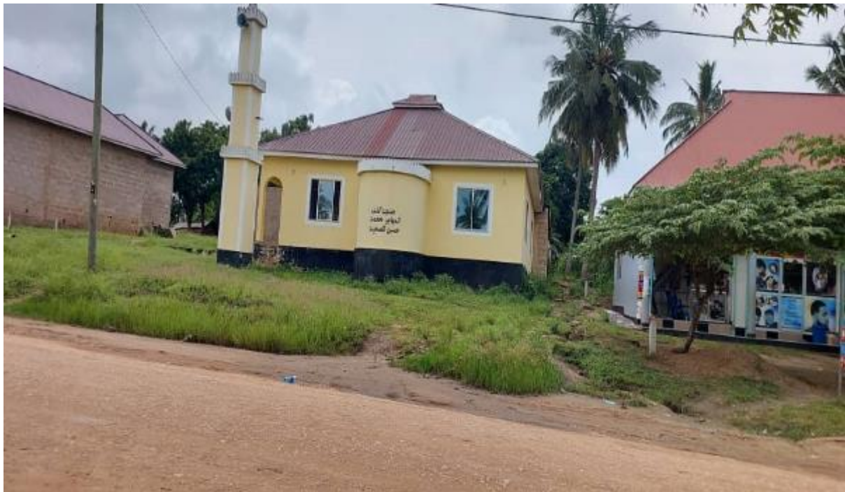
Figure 2-24: A Mosque at Km 5+ 100 LHS, beyond the Construction Corridor of the Proposed Goba-Wakorea Road
