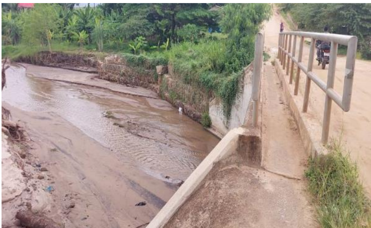
Figure 2-31: Msumi River Crossing the Road at Km 0 + 900
