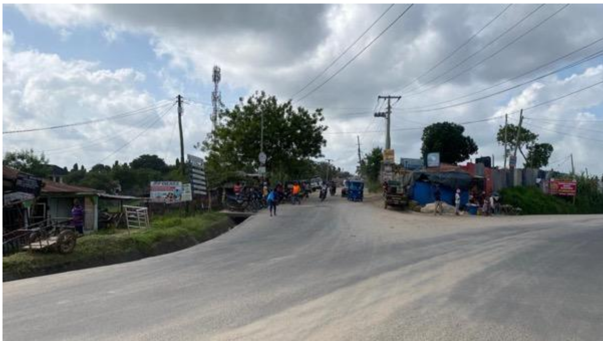
Figure 2-6: Start of Msumi Road at Junction of Njia Panda Makabe/Goba
