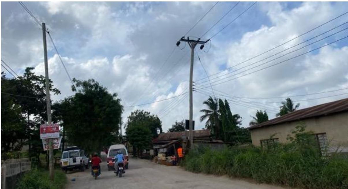
Figure 2-8: Residential Houses at Km 0 + 100 of the Proposed Msumi Road
