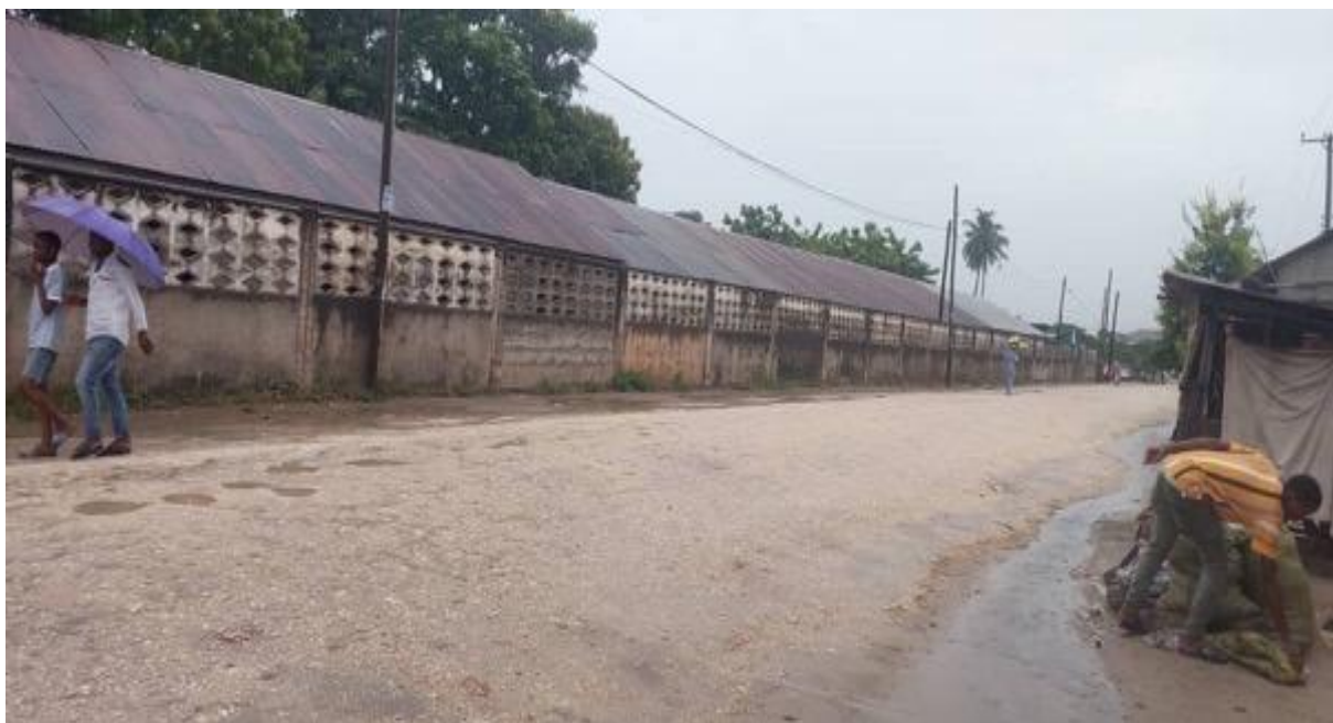
Figure 2-156: Compound Fence of Kawawa and Amani Primary Schools at Km 1+000 LHS of Binti Kayenga Road
