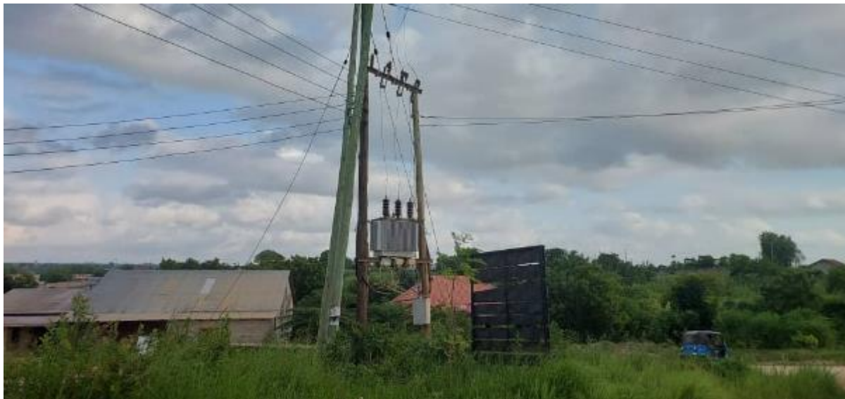
Figure 2-47: A Concrete Marker Post for Telecommunication Cable found at Km 0 + 600 RHS of the Proposed Hondogo Shija Road
