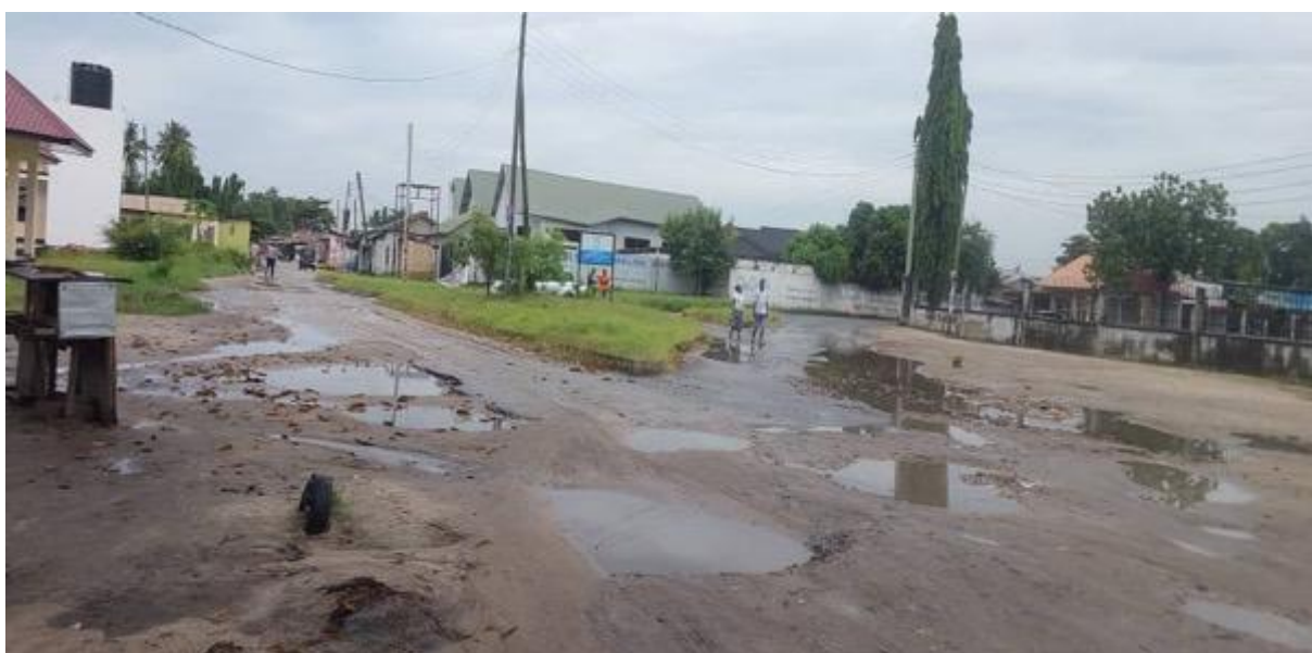
Figure 2-123: Starting Point of Ubungo NHC Road, an extension with Existing Tarmac Road Source: Field Survey by the Consultant (June 2023)
