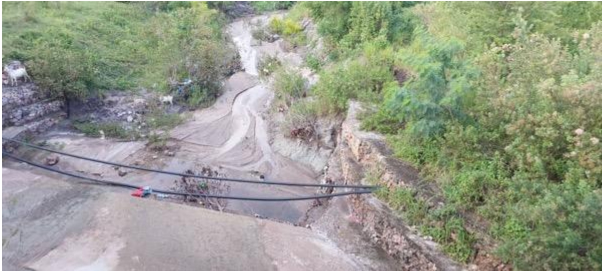
Figure 2-40: One of Lowest Point of Hondogo Shija Road: Kibwegere Seasonal River at Km 3+400
