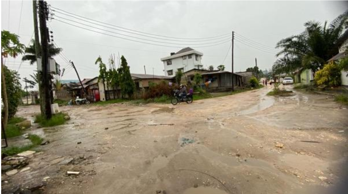
Figure 2-107: Starting Point of Mikindani Road, at Intersection with Mbegani Road
