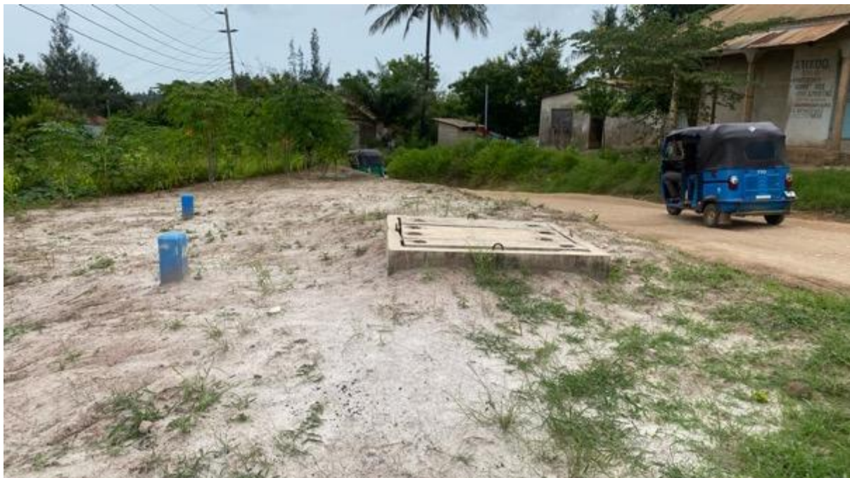
Figure 2-36: Water Supply Infrastructure within Road Construction Corridor at Km 0 + 500 LHS of the Proposed Goba-Wakorea Road
