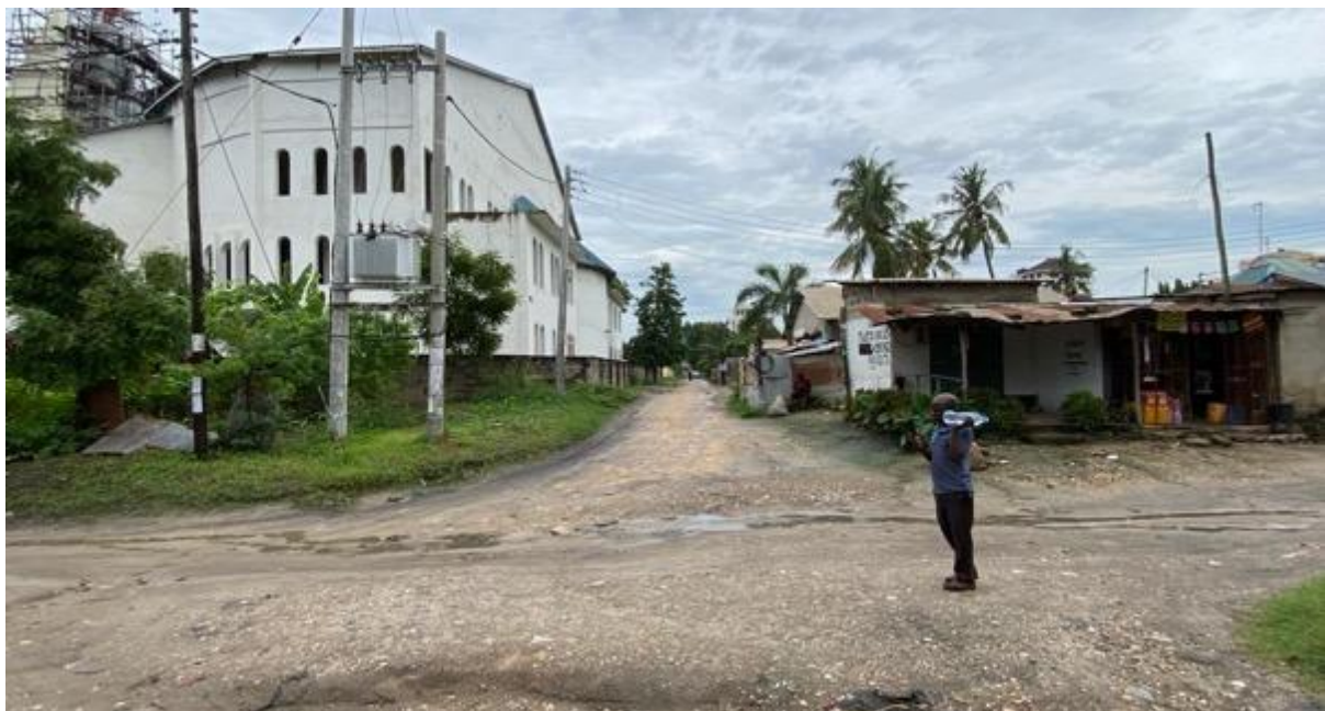
Figure 2-133: Electric Substation found at Km 0+150 of Ubungo NHC Road
