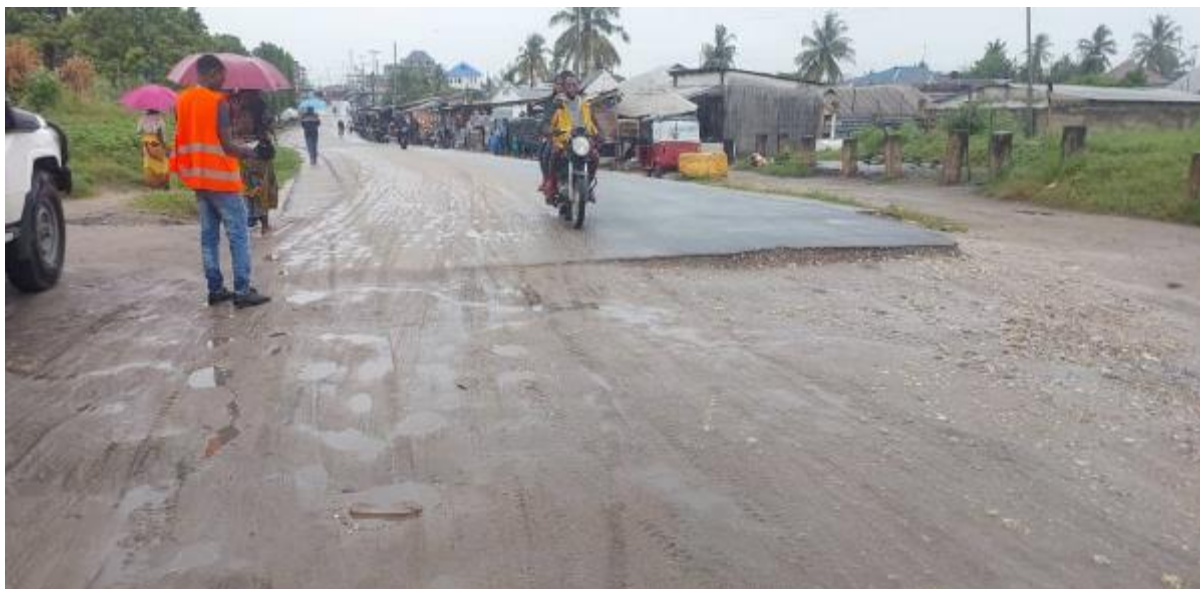
Figure 2-135: End Point of Tiptop Road, where it Meets Existing Tarmac Road to BRT Infrastructures of Morogoro Road
