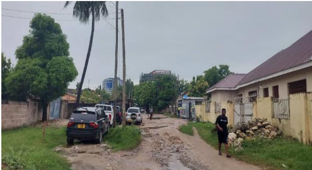
Figure 2-85: Electric Poles found at Km 0+090 of Segesera Road
