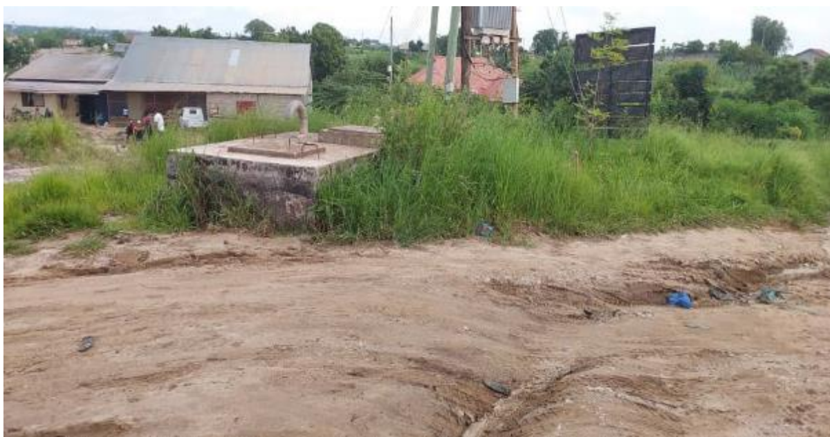
Figure 2-48: A Concrete Marker Post for Telecommunication Cable found at Km 0 + 600 RHS of the Proposed Hondogo Shija Road
