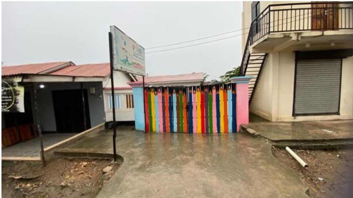
Figure 2-118: Power Day Care Nursery School found at Km 0+040 LHS of Lion Road
