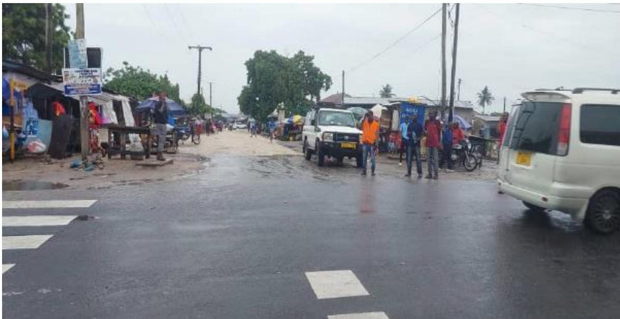
Figure 2-152: End of Binti Kayenga Road, a T-Junction with Kigogo Regional Road
