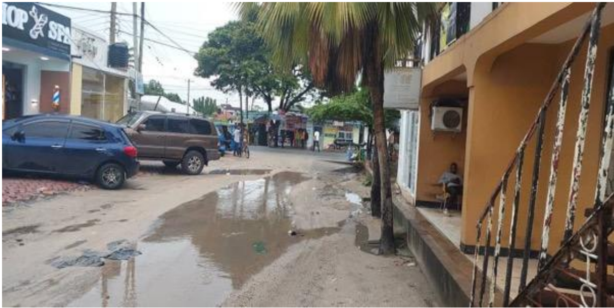
Figure 2-78: End of Segesera Road, a T-Junction with Sinza Mori Road
