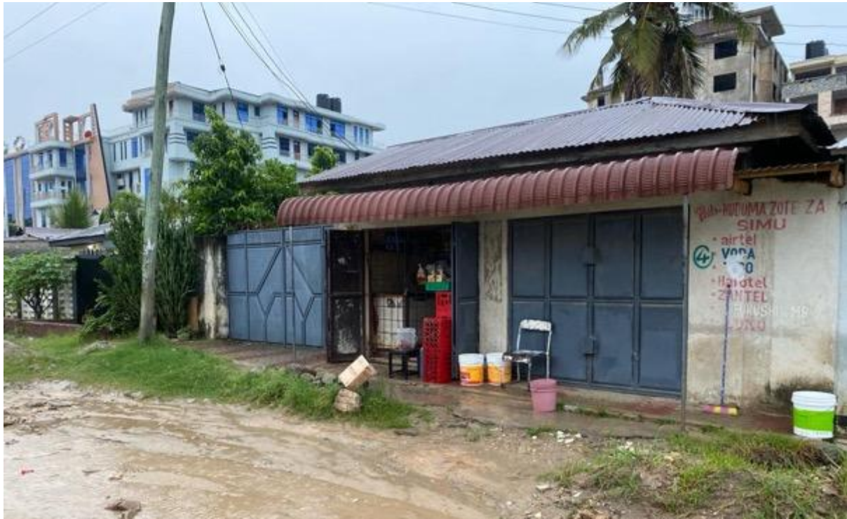
Figure 2-109: Shops at Km 0+060 LHS of Mikindani Road
