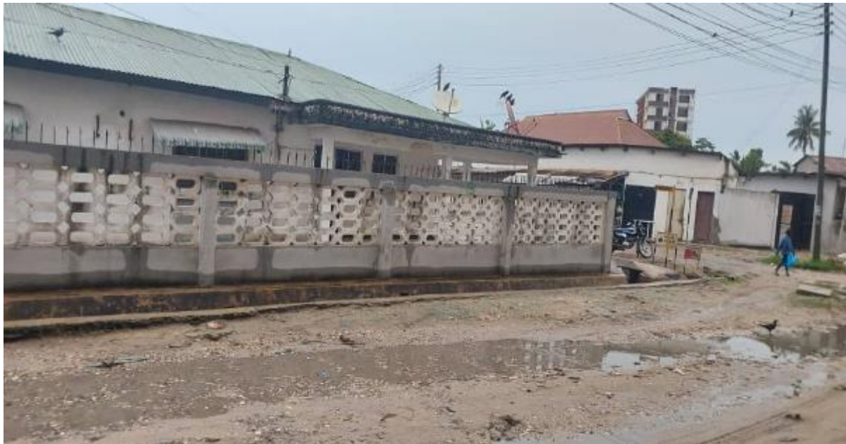
Figure 2-81: One of the Houses whose Fence will be Demolished, Photo Taken at Km 0+260 LHS of Segesera Road
