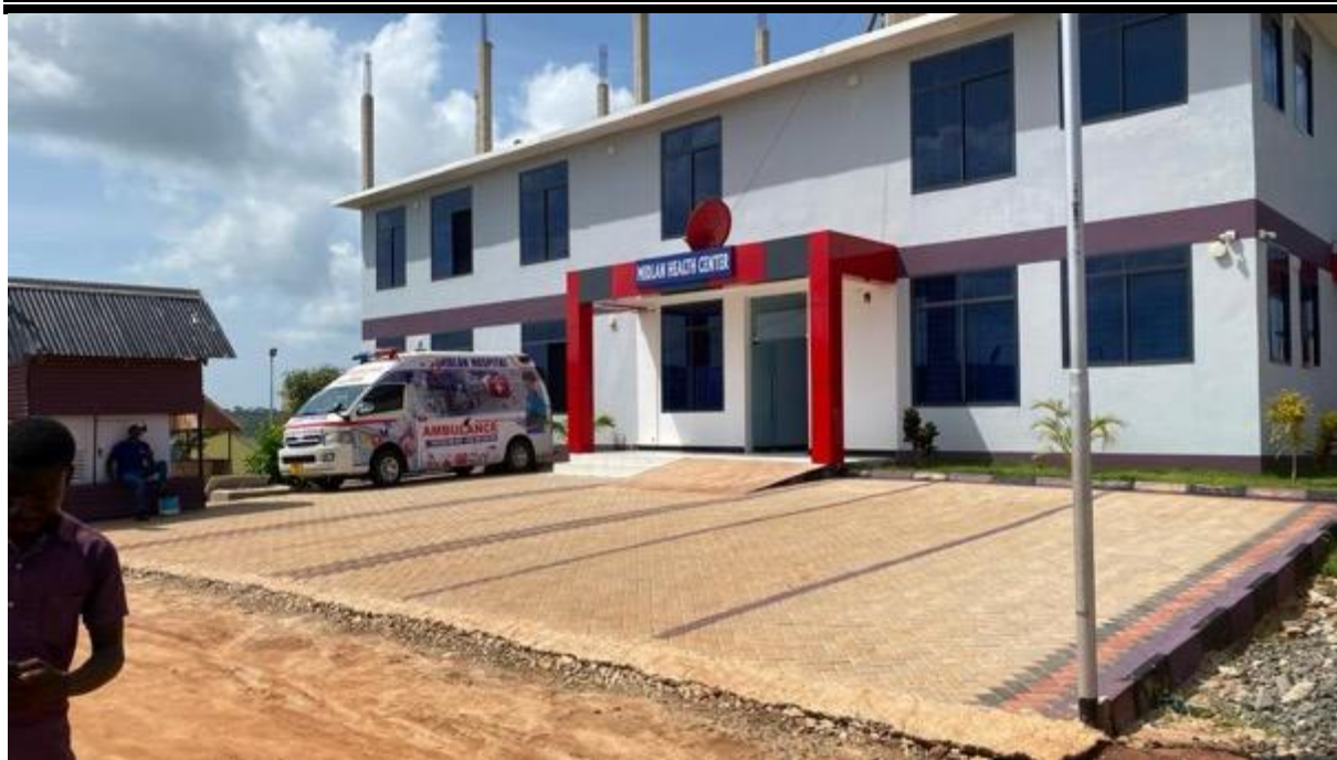
Figure 2-11: A Health Facility (Midlan Health Center) found at Km 6 + 700 LHS of the Proposed Msumi Road
