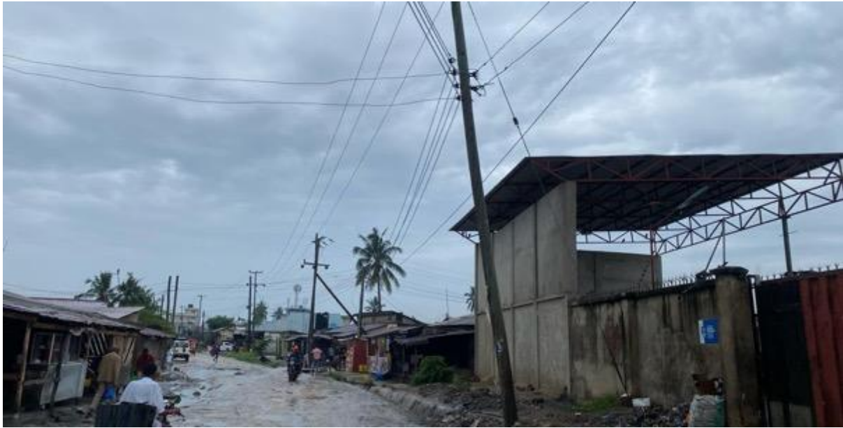
Figure 2-159: Electric Pole with Power Distribution Line at Km 0 + 100 LHS of Binti Kayenga Road
