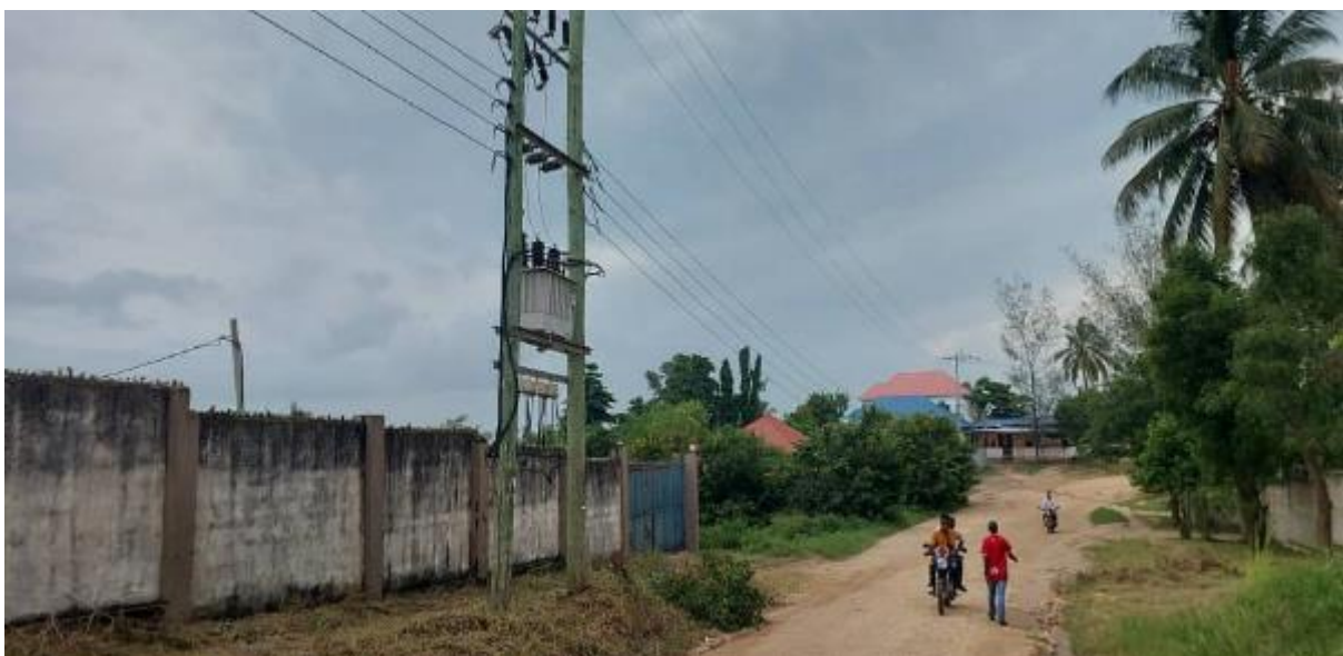
Figure 2-35: Electrical Power Line within Road Construction Corridor at Km 0 + 300 LHS of the Proposed Goba-Wakorea Road
