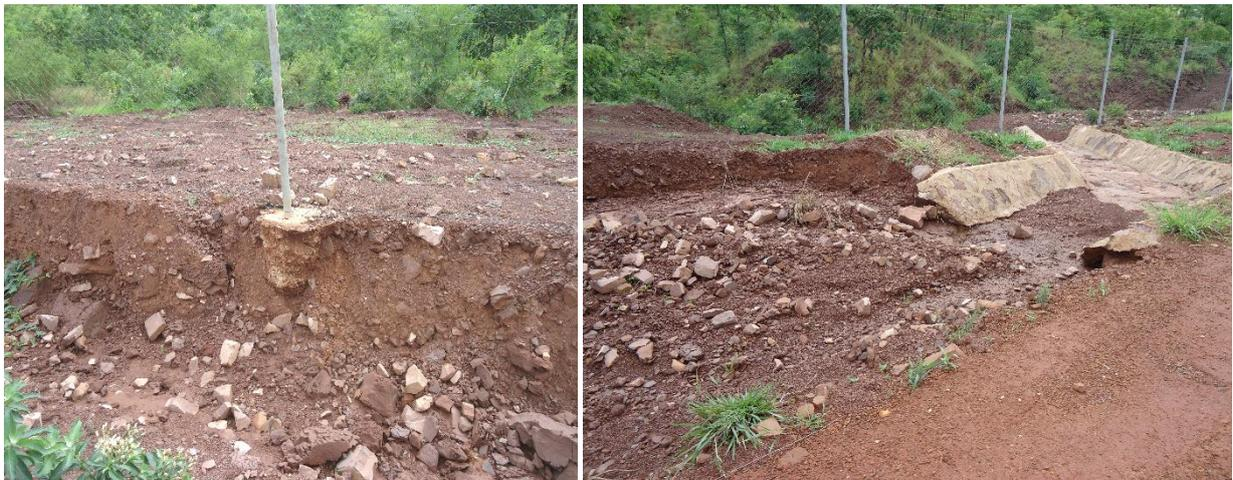
*Figure 4.9: The eroded fencing poles (L) and storm water drains (R) at the Msimba landfill*
