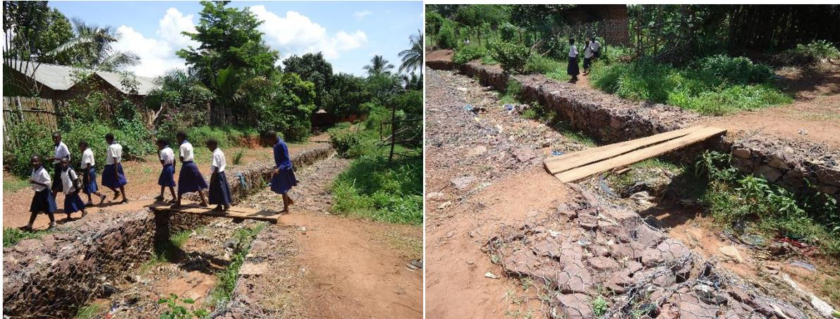
*Figure 4.5: Wooden planks used to cross over NHC-Katubuka drain*
