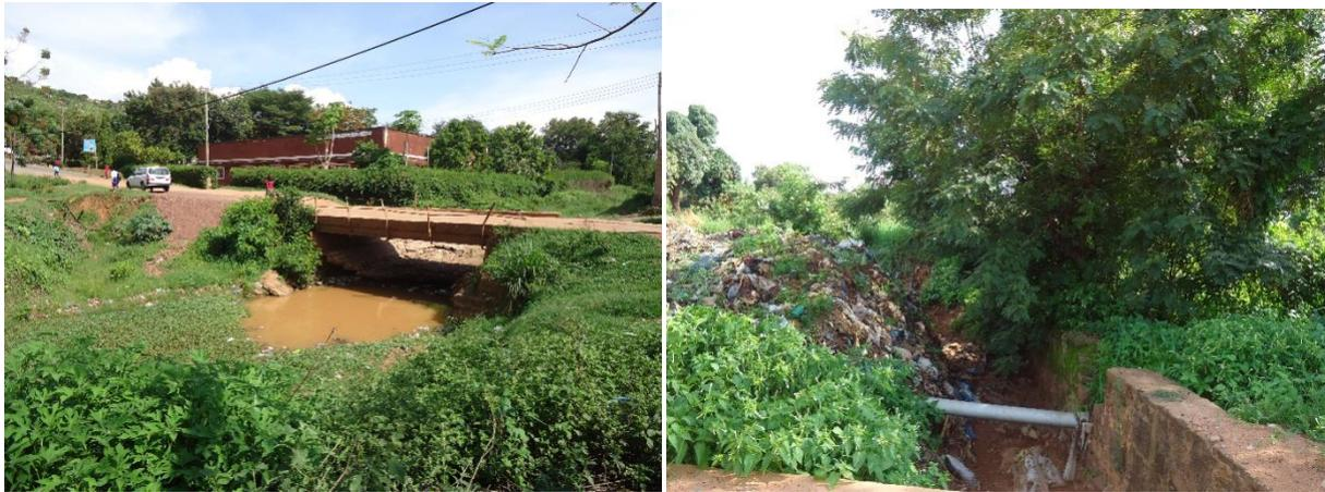
*Figure 4.4 Accumulation of silts (L) and solid waste disposal (R)*
