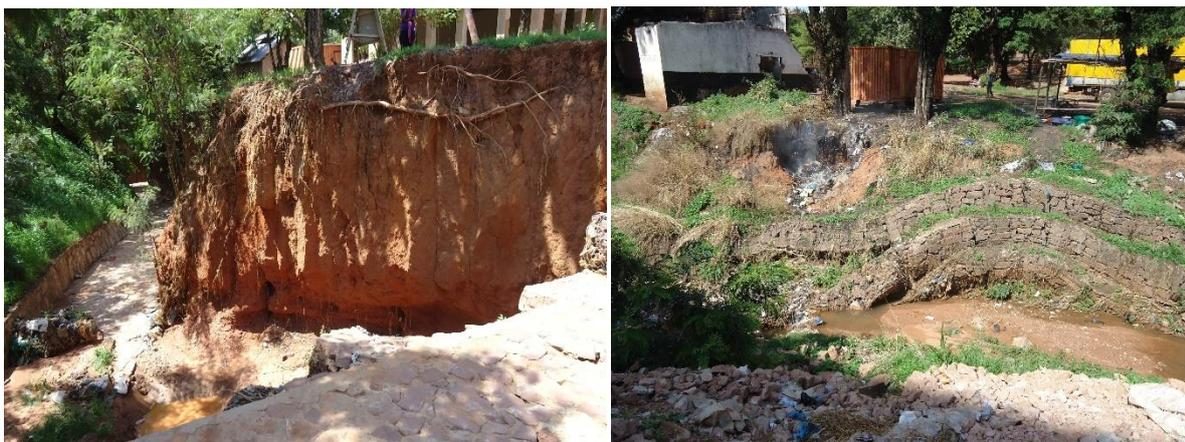
*Figure 4.3: Erosion (left) and destroyed gabions (right) along Lubengera drain*
