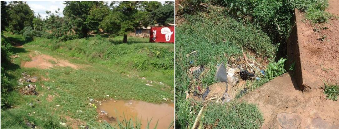
*Figure 6.2: Siltation of Lubengere (L) and NHC-Katukuka (R) drains*
